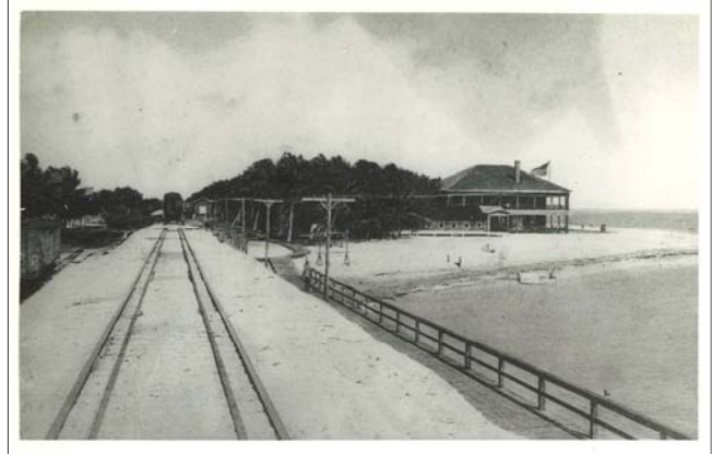
The Long Key Fishing Lodge as seen from the Long Key Viaduct.
